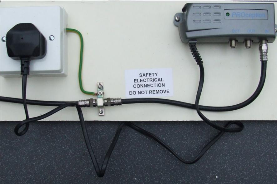
When the amplifier has no earth tag then use an earth connector block
