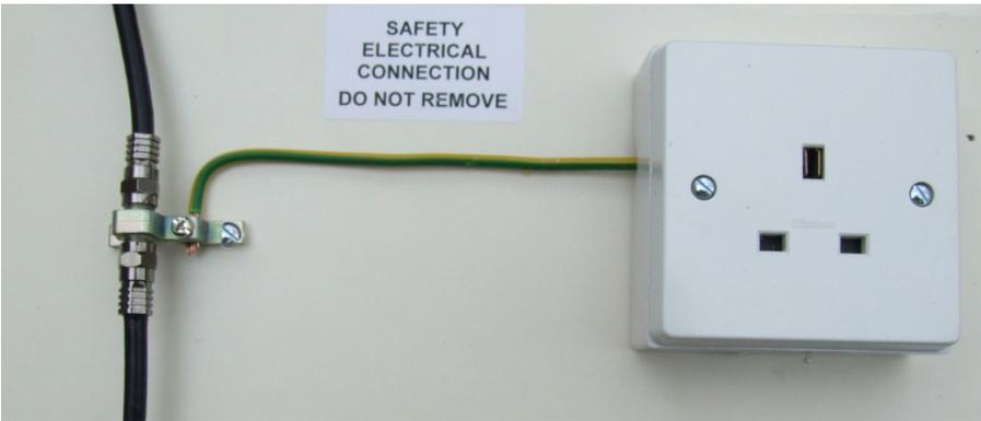
In a situation, such as when using an external amplifier or if no earth can be located near to the distribution point, the earth could be taken off the socket behind a TV for example.
