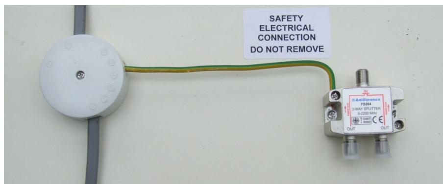
A simple connection off a lighting circuit junction box onto a passive device.
